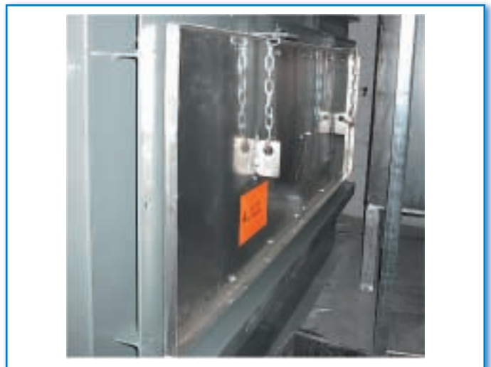
Explosion Relief Panel Designed and manufactured to meet specific NFPA requirements
