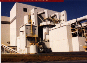
Wheelabrator NO x OUT system keeps nitrogen oxide emissions below 100 ppm from two 750-ton-per-day municipal solid waste incinerators in Morrisville, PA.
