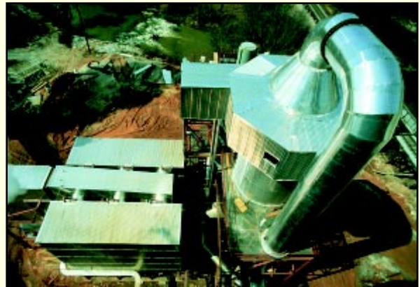
Emissions from a pulverized coal boiler.
