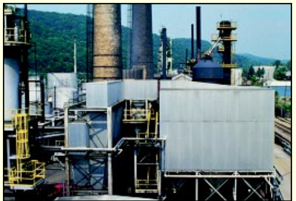
Emission from coal-fired boilers at an oil refinery.
