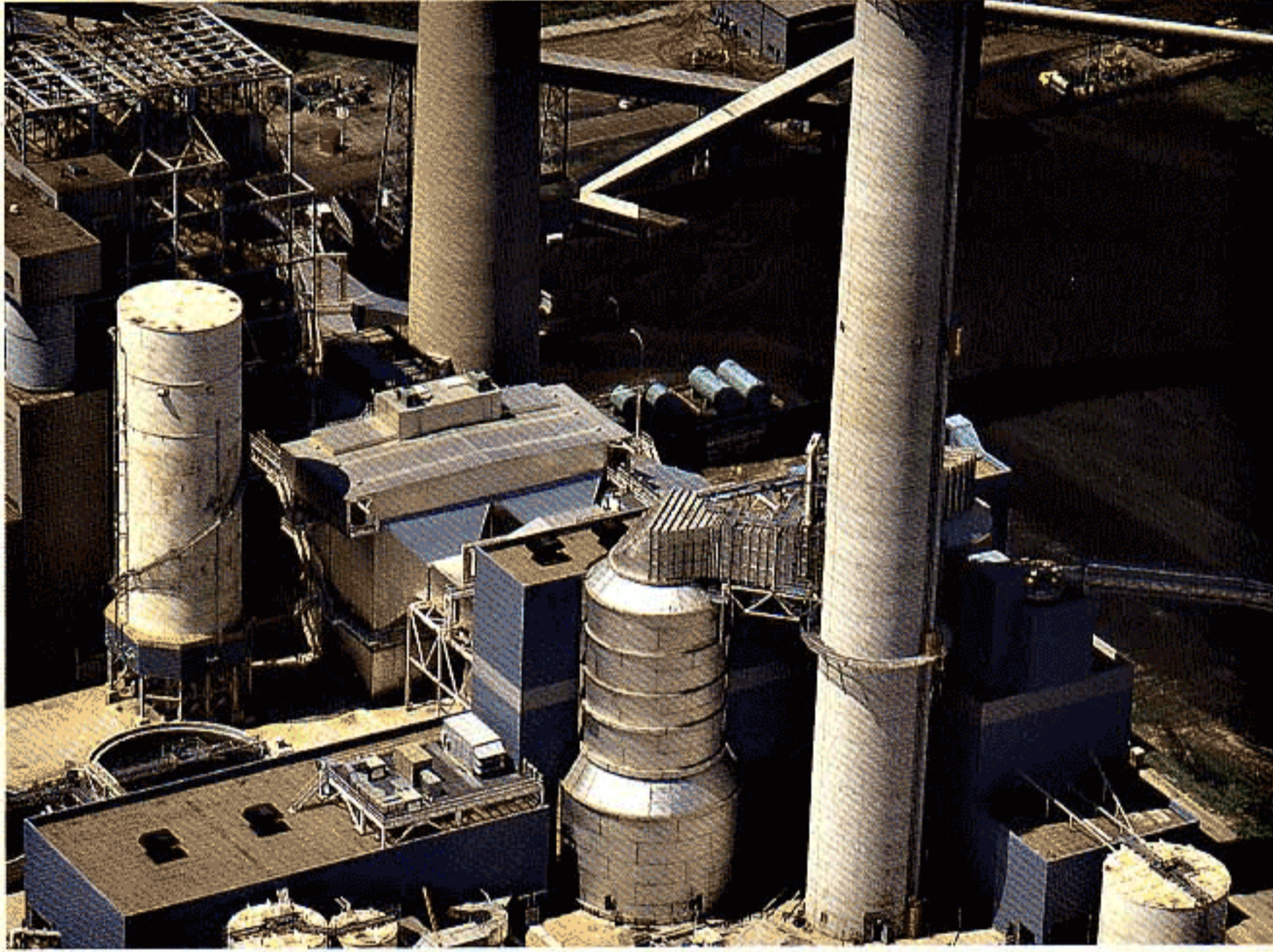
Wet open-spray-tower absorbers and electrostatic precipitators control SO 2 and particulate emissions from two coal-fired boilers at a 440 megawatt power plant in Owensboro, Kentucky.
